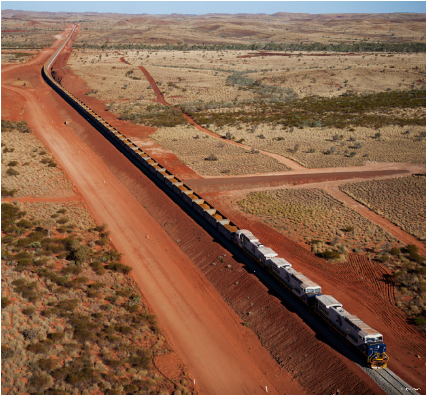
An Outback freight train takes iron ore to Port Hedland from Fortescue Metals Group's Cloudbreak mine in the Pilbara, Western Australia. Transport infrastructure associated with mining in Outback areas, such as road networks and rail lines, can increase the impact of industrial activity on the broader landscape.
