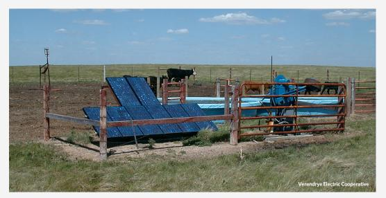
Solar-powered pumps for stock tanks.
