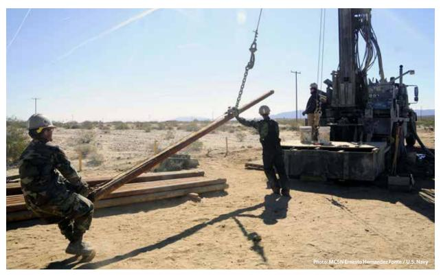
U.S. Navy Construction Electrician 3rd Class Robert Schiller, left, and Construction Electrician Constructionman Greg Langdon add a new section of drill steel to a T2W Ingersol-Rand Water Well-Drilling Rig in Twentynine Palms, CA, in 2009. Seabees from Naval Mobile Construction Battalion 1 drilled three 800- to 1,000-foot holes in the area to assist the U.S. Navy Geothermal Program Office in their research of local geothermal energy potential.
