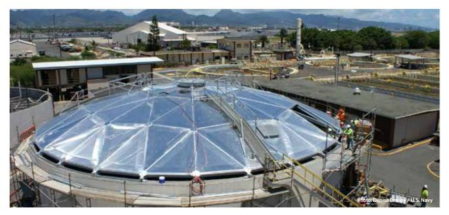
Naval facilities engineering teams upgrade the wastewater treatment plant at Joint Base Pearl Harbor-Hickam in Hawaii by replacing the floating steel roofs with fixed aluminum dome covers in 2011. The new covers help capture methane gas for future energy projects and for use as an alternative fuel source.
