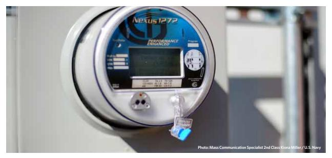
An advanced metering infrastructure smart meter is shown near the Catering and Conference Center at the Washington Navy Yard, DC, in 2011. The smart meter records energy consumption data every 15 minutes and sends the information to a single, secure system. The meters are intended to enable managers to monitor and control energy systems throughout the installation.
