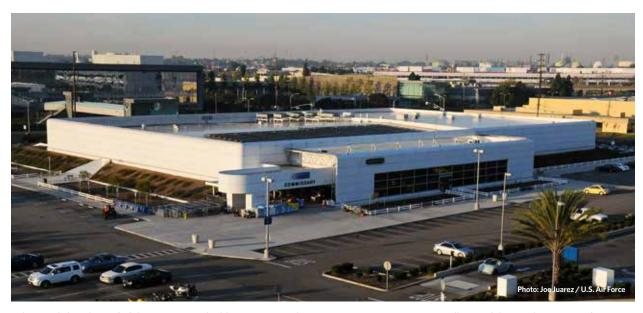
Solar panels line the roof of the commissary building at Los Angeles Air Force Base, CA, in 2011. Installation of the panels was part of ongoing energy conservation efforts on base.
