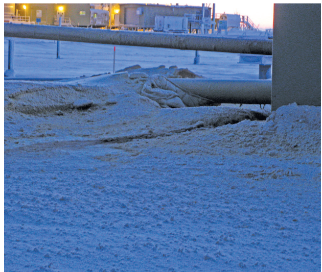
Dec. 23, 2009: Contaminated snow at the BP spill site in Prudhoe Bay after release of crude oil and produced water. A flow line is blamed.
