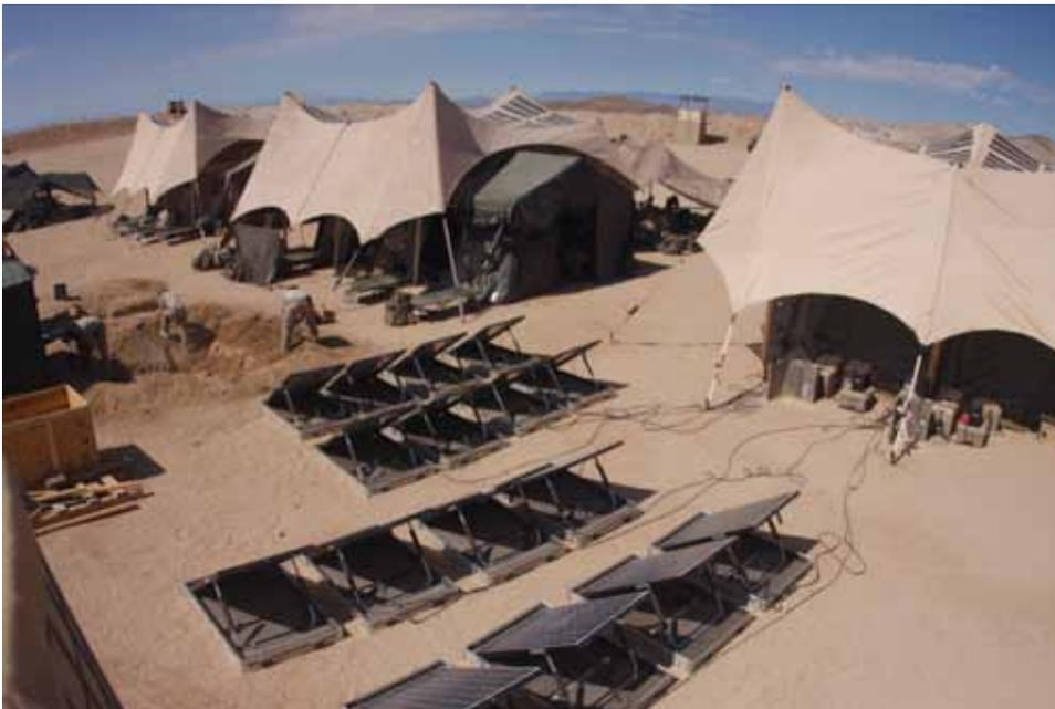
**POWERSHADES FIT OVER STANDARD MARINE CORPS TENTS AND CUT THE TEMPERATURE INSIDE BY 10-15 DEGREES. SOLAR PANELS EMBEDDED INTO THE CANVAS PROVIDE ENOUGH ENERGY TO RUN THE TENT'S LIGHTS.**
