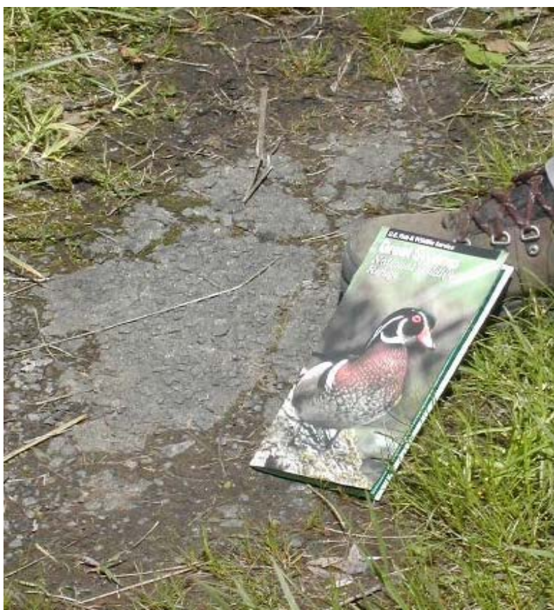
This May 2002 photo along the former road right-of-way within the Great Swamp Wilderness shows a small patch of road surface missed during the removal work 30 years earlier
