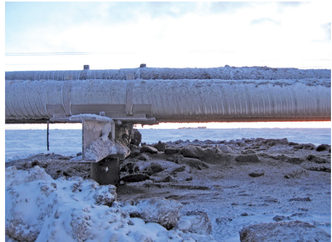
Dec. 1, 2009: Area of heaviest contamination mounded below spill site. Photo: ADEC
