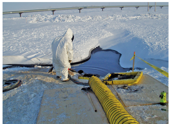
March 3, 2006: Cleanup of GC-2 oil spill that released 212,000 gallons of crude oil in the largest spill on the North Slope. Oil spilled from a quarter-inch hole in the pipeline, caused by corrosion. Nearly two acres of tundra and frozen lakes were impacted.
