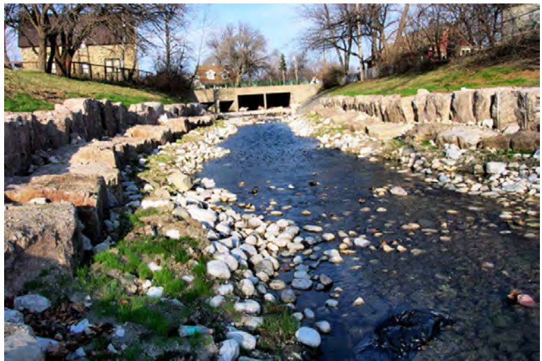
Rocks, grass, and native vegetation bordering Milwaukee's Lincoln Creek allow rainwater to soak into the ground. The creek used to be lined with concrete, and it flooded more than 4,000 times before the human-made material was replaced with natural buffers. Milwaukee Metropolitan Sewerage District
