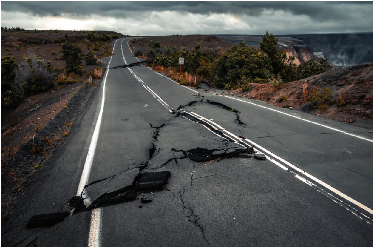
The asphalt in a road cracked open after the 2018 eruption of the Kilauea volcano in Hawaii's Volcanoes National Park, which was followed by some 60,000 earthquakes. Work on repairing the damage—including collapsed roads, toppled buildings, rock falls, and breaks to water and sewer lines—continues to this day. Dudarev Mikhail/Shutterstock
