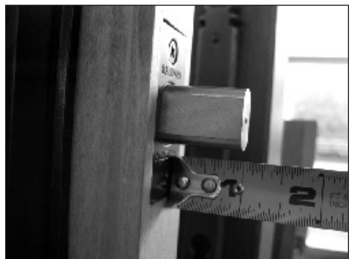
Exterior doors should have deadbolts as a form of access control. The deadbolt’s “throw” should be at least 1 inch, making the door harder to kick in.
