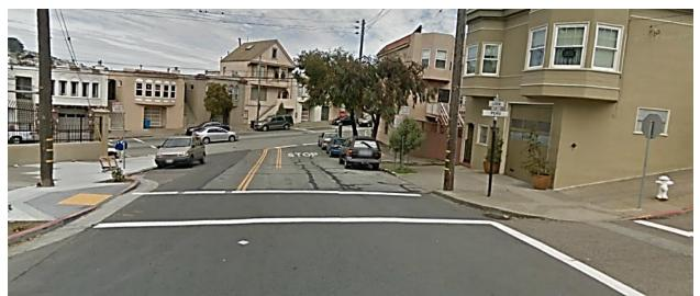
Figure 5. Lisbon Street and Peru Street: absence of a curb ramp at a marked crosswalk. Source: Google StreetView
