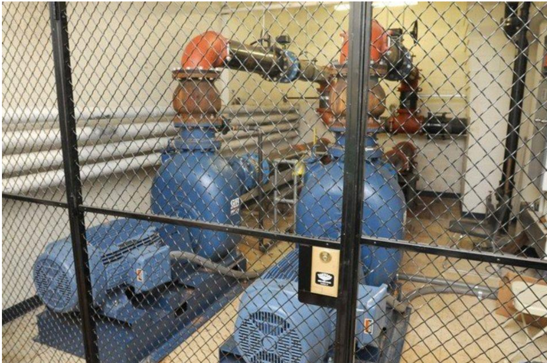
Figure 2. The stormwater pump stations at Gerena Community School (photo by Mark Murray from a February 9, 2012 article in the Republican).
