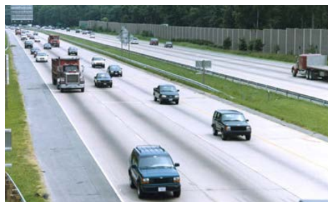
Figure 37: Noise Barrier that Reduces Noise Impacts to Surrounding Areas Source: VDOT
