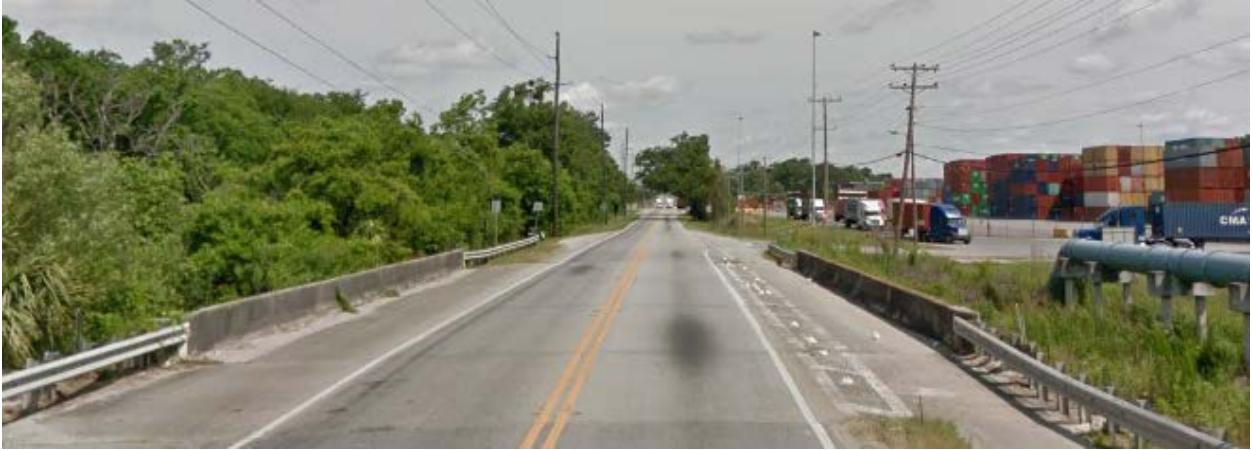
Figure 17: State Route 25 at Pipemaker Canal Source: Google Streetview, 2016
