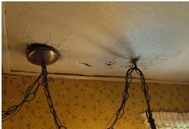
Image 2: Water and roof damage
