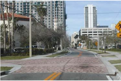
Speed table Photo courtesy of FHWA.
