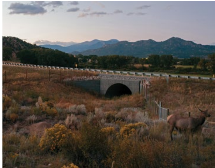
An elk (foreground, right) stands beside fencing that helps direct animals to an underground crossing tunnel on U.S. 285 near Buena Vista, Colorado. Structures built under or over busy roads help animals to safely navigate traditional migration routes while also reducing traffic collisions.
