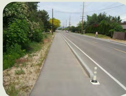
Left: An extruded curb with a shoulder provides a flat walking area in situations where sidewalk installation is cost-prohibitive.
