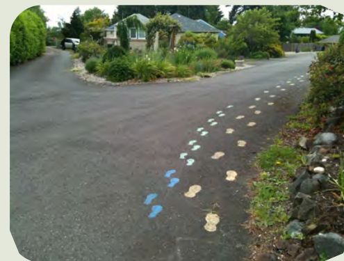
Left: Pedestrian shared lane markings are an innovative treatment to simply raise the awareness of pedestrians on a residential street. They are simply feet or shoe markings painted on one side of the street.
