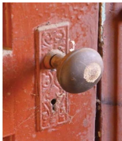
The current interior conditions at 493-A Auburn. NPS estimates that the unit still needs $259,889 to restore the interior, which retains many original historical features, such as moldings and fixtures. Interior conditions at 493-B and 493-C are similar.
