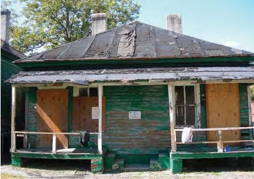
493-A Auburn Ave. as it appeared when it was acquired in very poor condition by NPS in 2003. 493-B and 493-C Auburn were in similar condition.
