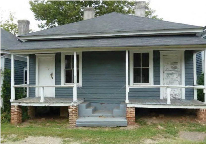
493-B Auburn (identical to 493-A) as it appeared in 2009 after emergency stabilization work was performed on all three properties.
