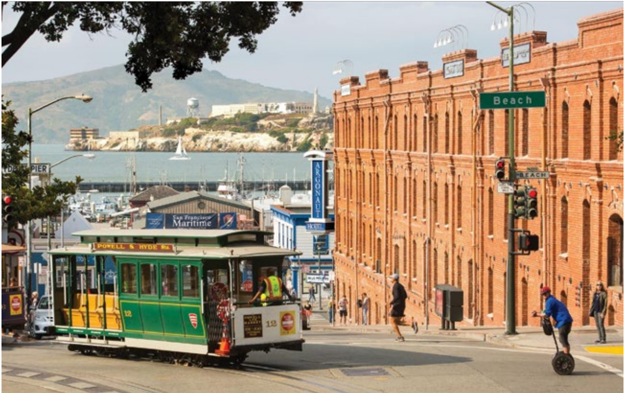
An expansive 100-year-old red brick waterfront building at the San Francisco Maritime National Historical Park has a new role. The former warehouse and cannery is now a boutique hotel, thanks to an innovative National Park Service leasing program. argonauthotel.com
