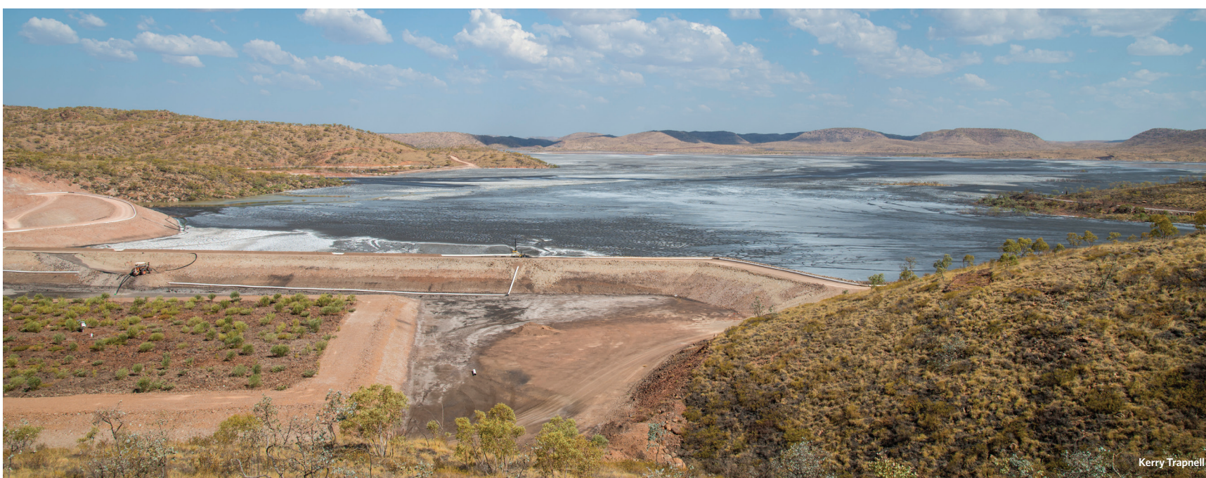
The tailings dam at Century Mine covers 376 hectares (top). MMG Limited hopes to extract zinc from sediments before rehabilitating the dam (bottom). A rehabilitation plan is currently being developed.
