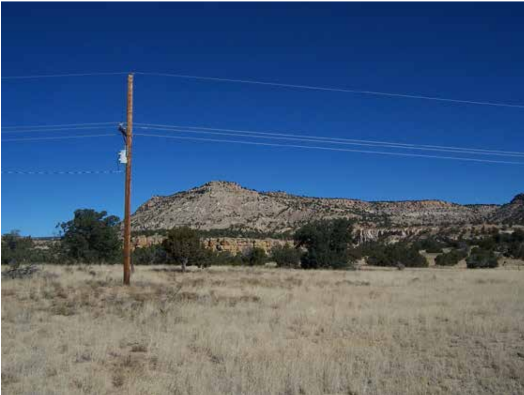
Figure 14. Power line crossing Section 16 portion of project site
