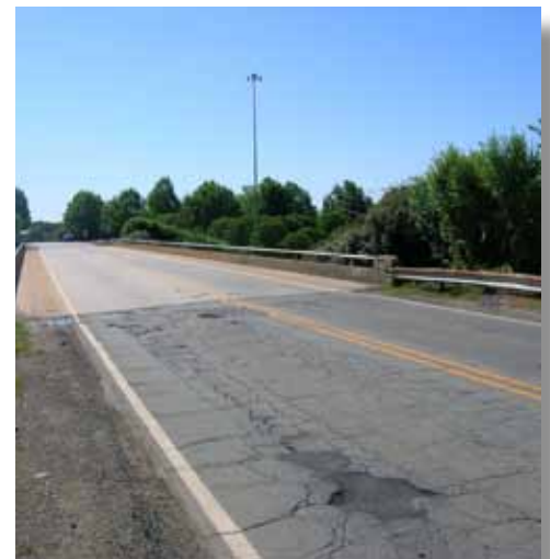
The I-77 bridge, exit ramps, and the adjacent section of Griffith Street are Bold Bicyclist streets due to high speeds, high traffic volume, and a lack of bicycle facilities.
