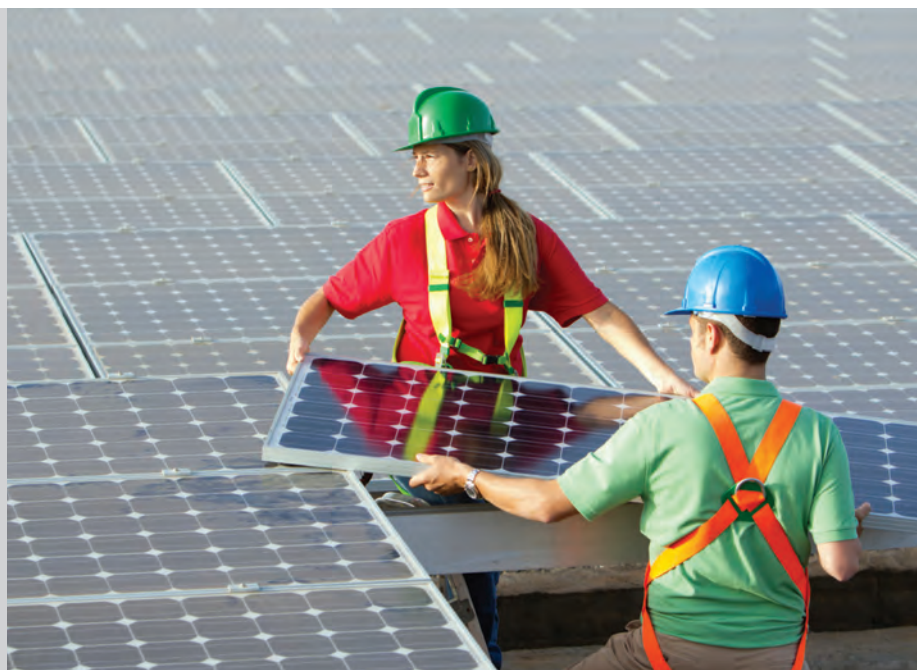
Two workers install a solar panel at a photovoltaic farm.
