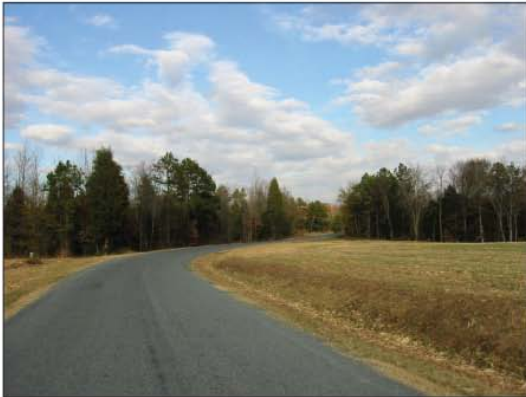
The photograph of June Washam Rd. shows a rural road that utilizes drainage swales instead of curb and gutter.
