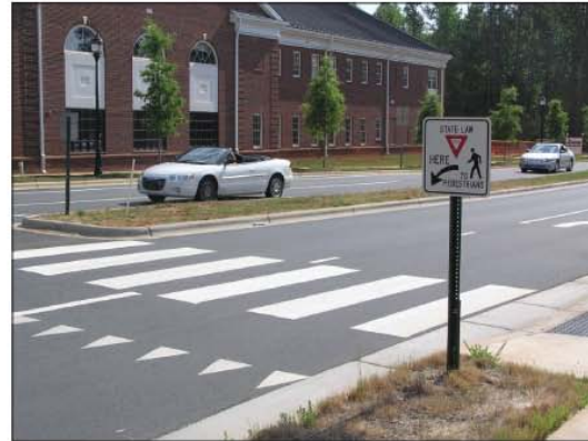
Streets become more pedestrian friendly by including crosswalks and a median refuge as shown above next to Davidson Day School on Griffith St.
