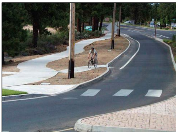
Bicyclist using exit ramp to access sidewalk prior to entering a roundabout.
