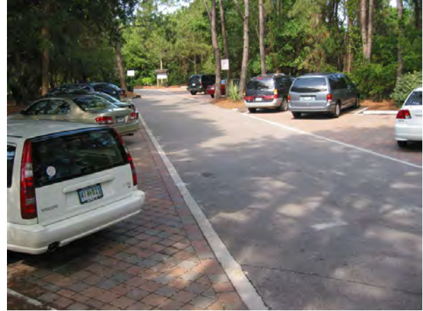
Figure 58. Example of permeable pavement parking. Credit: ICPI
