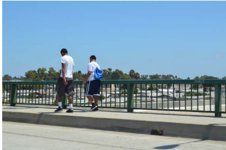
Figure 6-9. Pedestrians Using an Unprotected Sidewalk on an Arterial Crossing the Freeway
