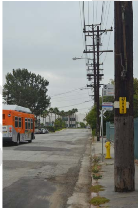
Figure 6-8. A Sidewalk at a Bus Stop that is Narrow and Has Many Impediments to Walking
