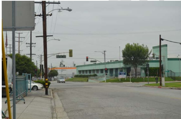
Figure 6-10. An Intersection in a Commercial Neighborhood with Poorly Marked Pedestrian Crosswalks, No Pedestrian Signals, and Impediments in the Surrounding Sidewalks
