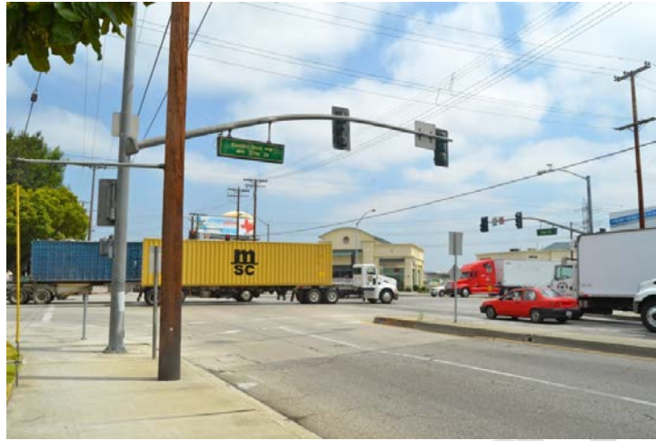
Figure 6-11. A Second Example of an Intersection in a Commercial Neighborhood with Poorly Marked Pedestrian Crosswalks, No Pedestrian Signals, Impediments in Surrounding Sidewalks, as well as High Volumes of Truck Traffic
