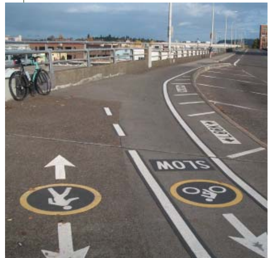
Bicycle and pedestrian facilities on bridge
