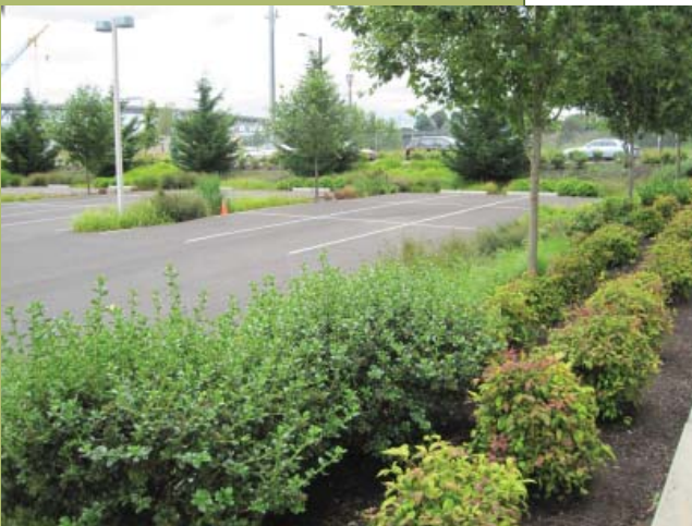
Low impact storm water facilities provides greenery in a parking area
