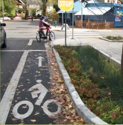
A complete street with bicycle facilities, sidewalks, and storm water facilities
