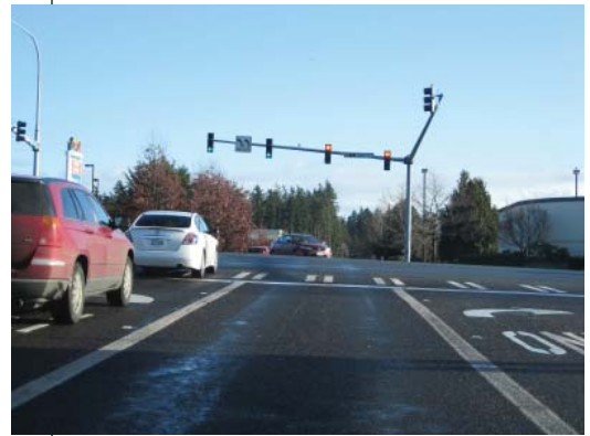
Large intersections and high vehicle speeds increase the need for safe pedestrian facilities
