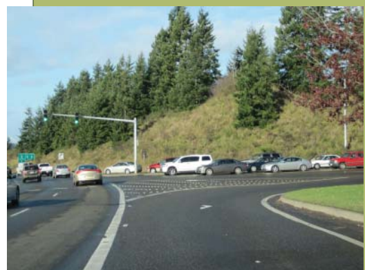
Meridian corridor approaching SR 512
