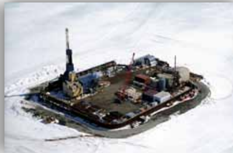
Figure 3-7. Example of Gravel Island-Based Production in Prudhoe Bay (Photos: BP)—The Northstar Unit (near left), operated by BP, produces from state and federal waters in the Beaufort Sea. The drilling operations are conducted from a five-acre
