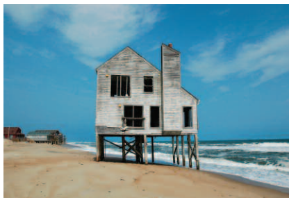
Erosion along Cape Hatteras, N.C., has been about 12 feet per year in recent years, leaving houses stranded. Common remedies—rebuilding structures and bulldozing sand back onto the beaches—actually increase erosion damage, according to scientists.
