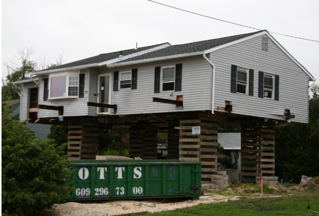
Home are being elevated
