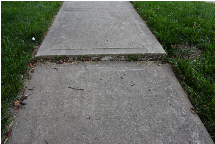
Image 6 – Picture of sidewalk needing maintenance
