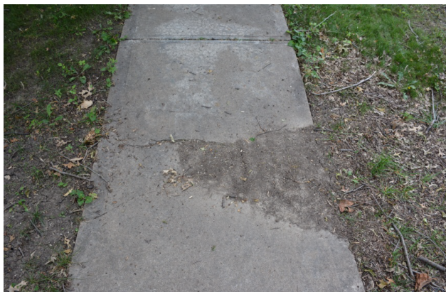
Image 5- Neighborhood sidewalk in disrepair
