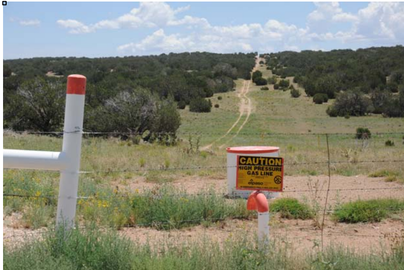
Figure 9. El Paso gas pipeline scar near Gran Quivira, east side of NM SR 55. July 2014.
