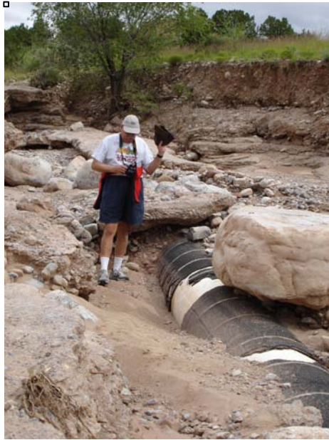
Figure 14. Excavation of 16/20-inch Enterprise natural gas pipeline by flood waters, Las Huertas Creek, 2006. Source: Las Placitas Association
