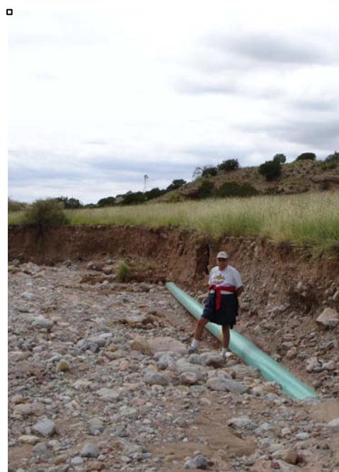
Figure 14. Excavation of 16/20-inch Enterprise natural gas pipeline by flood waters, Las Huertas Creek, 2006. Source: Las Placitas Association
