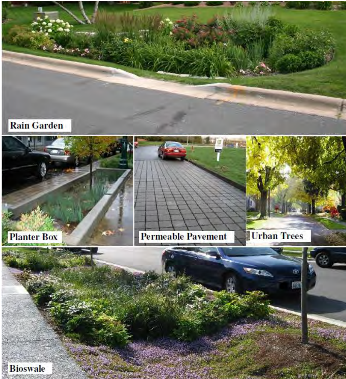
Figure 3. Examples of green infrastructure (U.S. EPA, 2014b).
