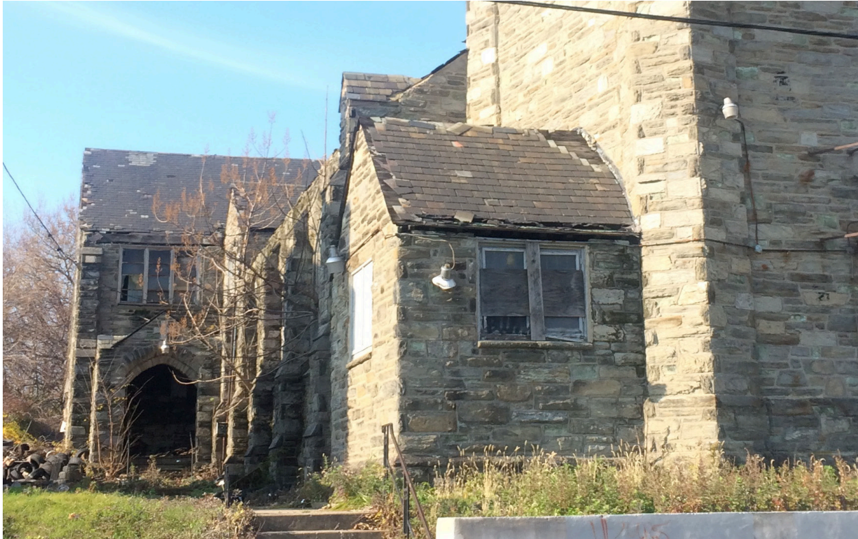
The former home of the Bethel Holy Temple Church in North Philadelphia sits vacant and in disrepair.
