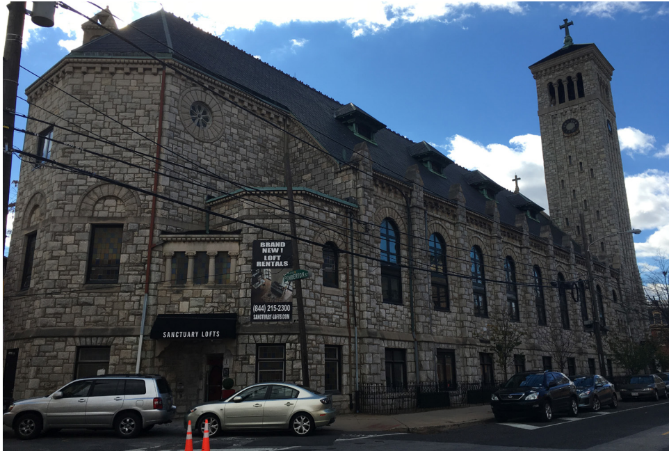
A 128-year-old church building in the Graduate Hospital neighborhood of Philadelphia is now Sanctuary Lofts, a multi-unit residential rental property that promotes itself as “the answer to your prayers.”
