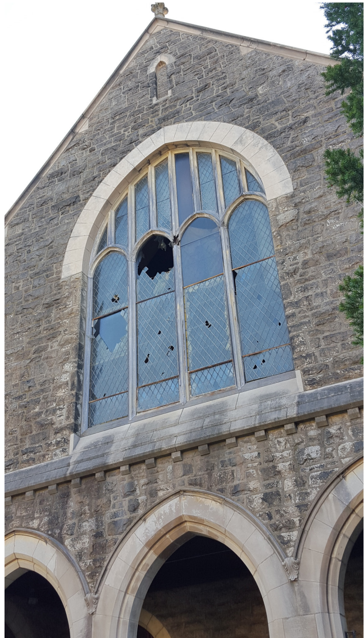
The vacant former home of New Covenant Baptist Church in Germantown shows signs of disrepair.
