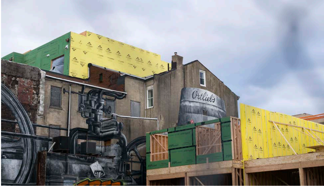
New construction on the site of the old Ortlieb's brewery in Northern Liberties, 2016.
