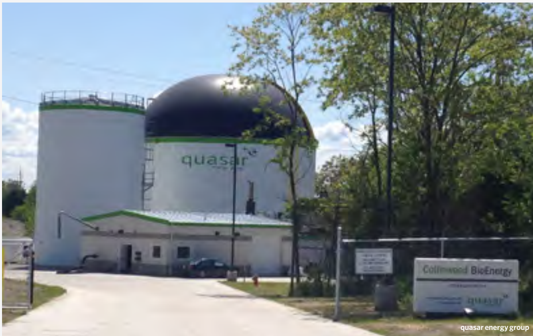
The 1-MW Collinwood BioEnergy facility, which converts sewage and food waste into electricity.
