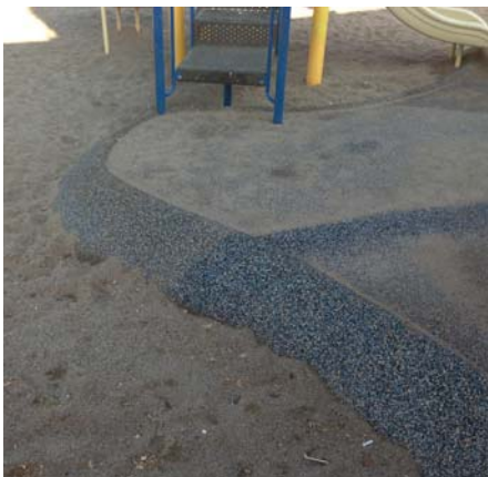
Low sand levels on playground
