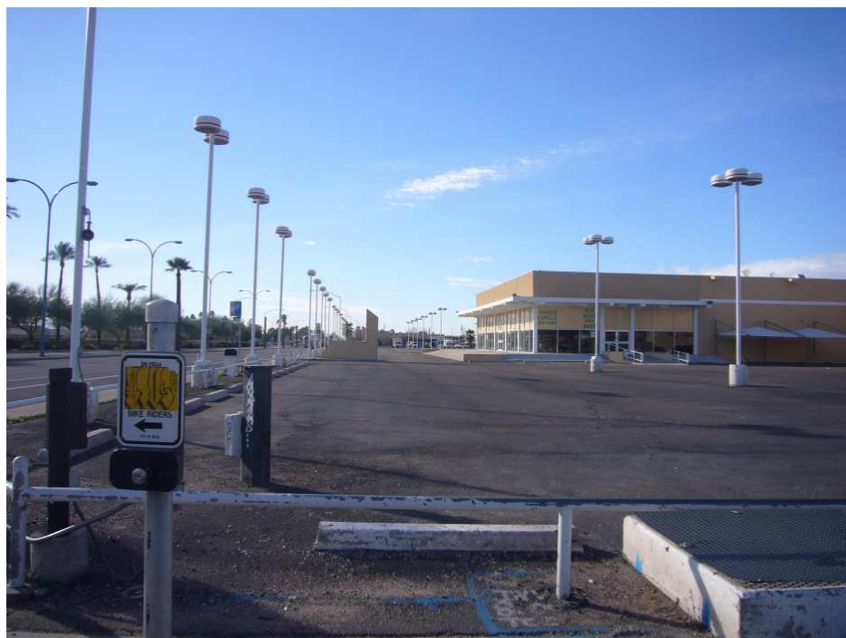
Figure 4.5.6 – Photo of 50's Era Commercial Building Stock With Excessive Asphalt Paving
