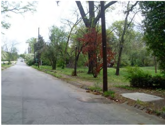
Figure 109: Lack of pedestrian facilities
