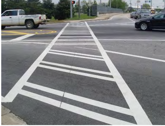
Figure 129: Pedestrian infrastructure does not reduce conflicts with turning cars and trucks
