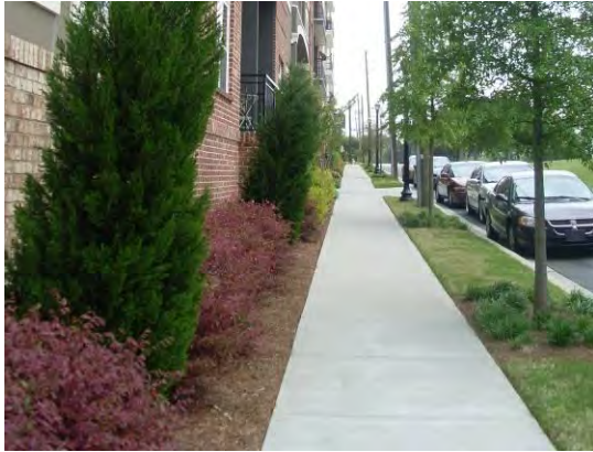
Figure 93: Attractive new infrastructure
