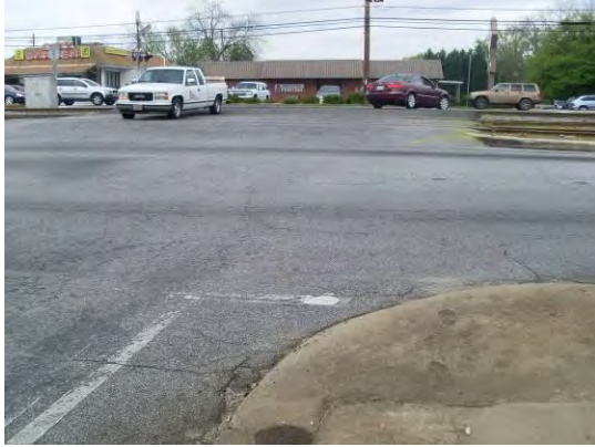
Figure 117: Lack of pedestrian infrastructure
