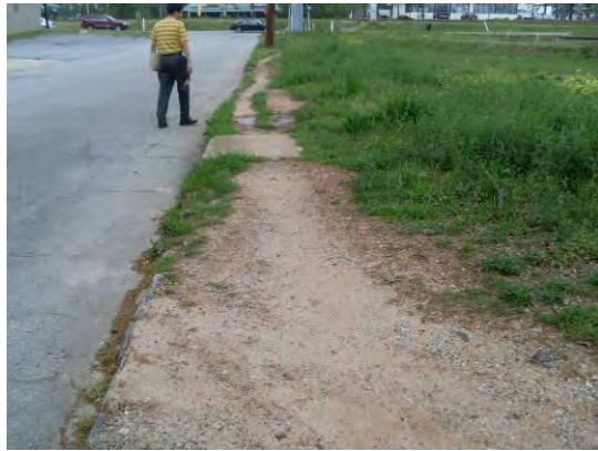
Figure 110: Lack of pedestrian facilities
