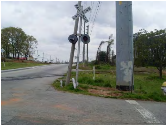
Figure 113: Lack of pedestrian infrastructure
