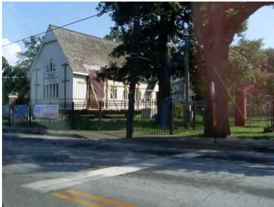
Figure 185: Pedestrians encounter varying roadside conditions
