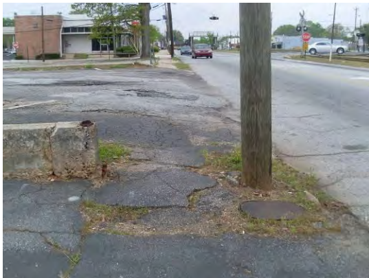
Figure 115: Lack of pedestrian infrastructure
