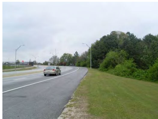
Figure 72: Absent sidewalks and crosswalks
