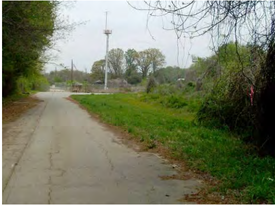
Figure 73: A neglected street
