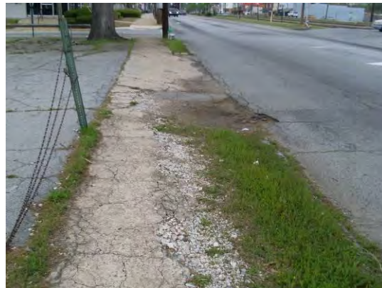
Figure 116: Lack of pedestrian infrastructure
