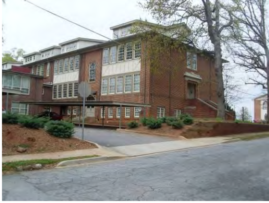
Figure 107: Condition of pedestrian facilities
