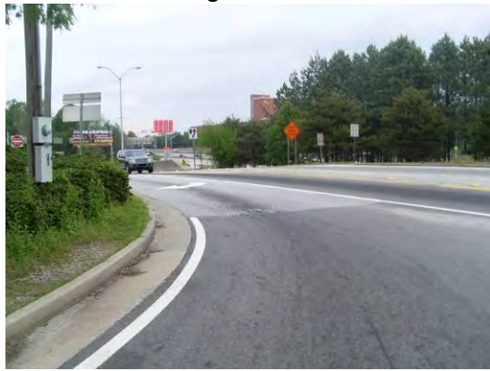
Figure 132: Pedestrian infrastructure does not reduce conflicts with turning cars and trucks
