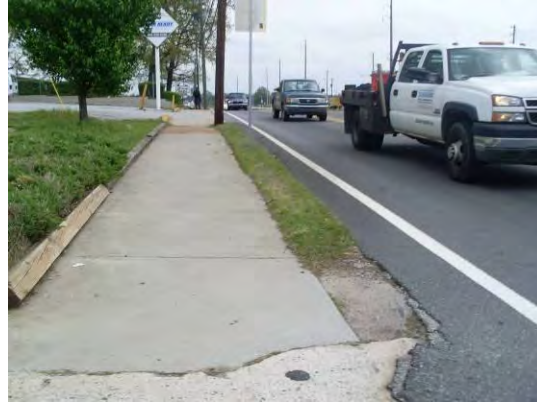
Figure 154: Proximity to traffic, pavement conditions
