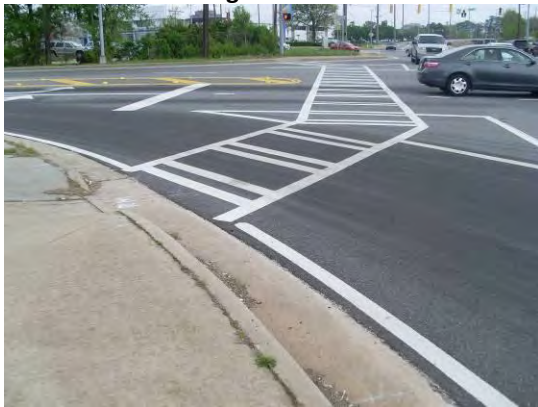
Figure 133: Pedestrian infrastructure does not reduce conflicts with turning cars and trucks
