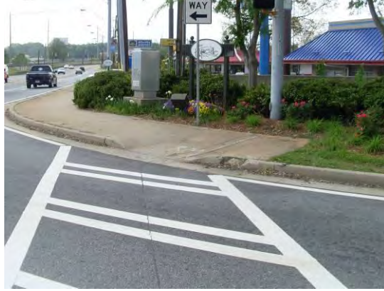
Figure 130: Pedestrian infrastructure does not reduce conflicts with turning cars and trucks
