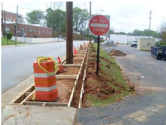
Figure 161: Some gaps in the walkway
