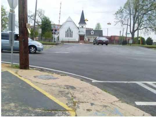
Figure 175: Some missing connections
