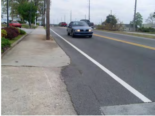
Figure 153: Proximity to traffic, pavement conditions
