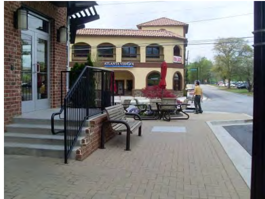
Figure 94: Attractive new infrastructure
