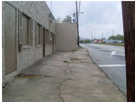
Figure 114: Lack of pedestrian infrastructure
