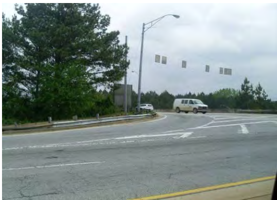
Figure 71: Absent sidewalks and crosswalks
