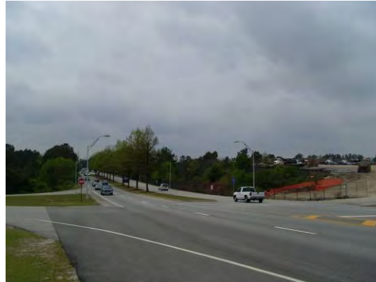
Figure 74: A neglected street
