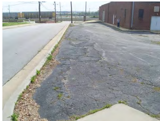
Figure 148: Broken or missing sidewalks
