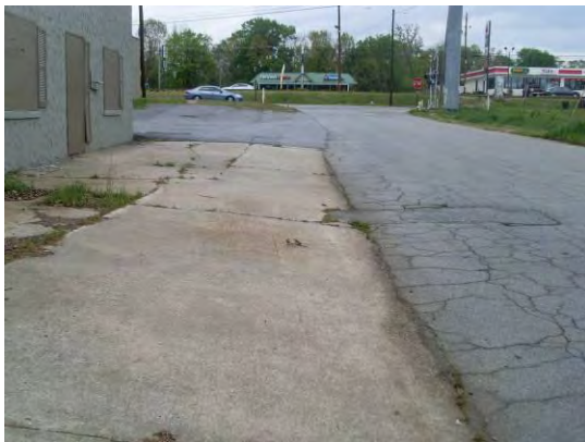
Figure 111: Poor condition of pedestrian facilities
