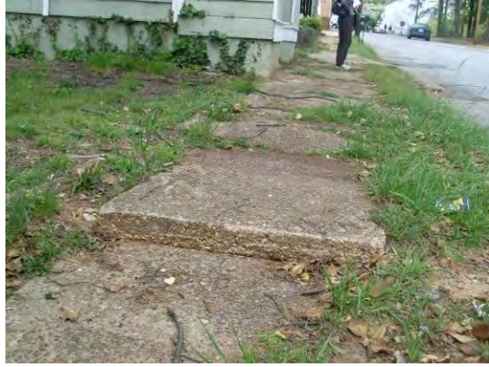
Figure 108: Condition of pedestrian facilities
