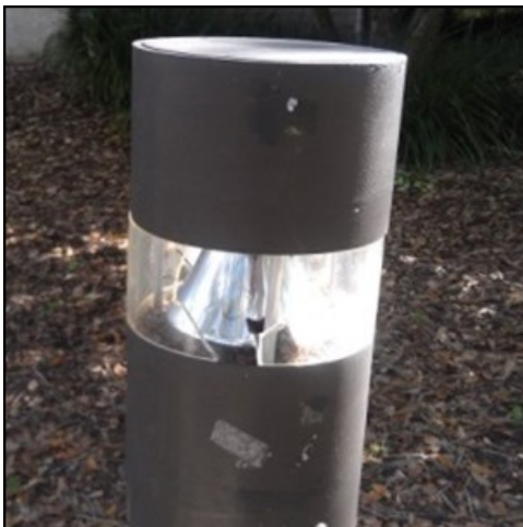
( Left ) View of one of the many weathered, damaged and outdated park light fixtures situated near a pathway.
