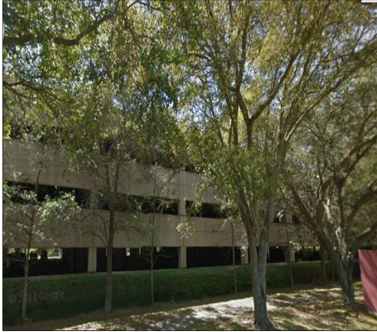
J: Multi-story Science Center Parking Garage located off Princeton St. The garage is connected to the Science Center via a walkway tunnel above the Princeton Street.
