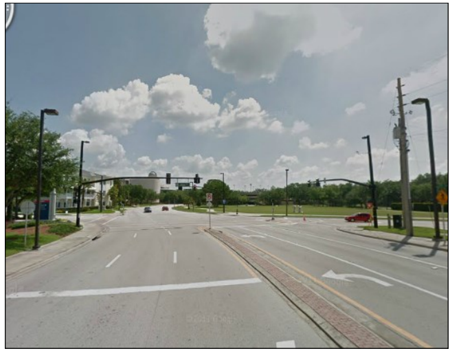
Looking east along Princeton at the intersection of Alden Road.
