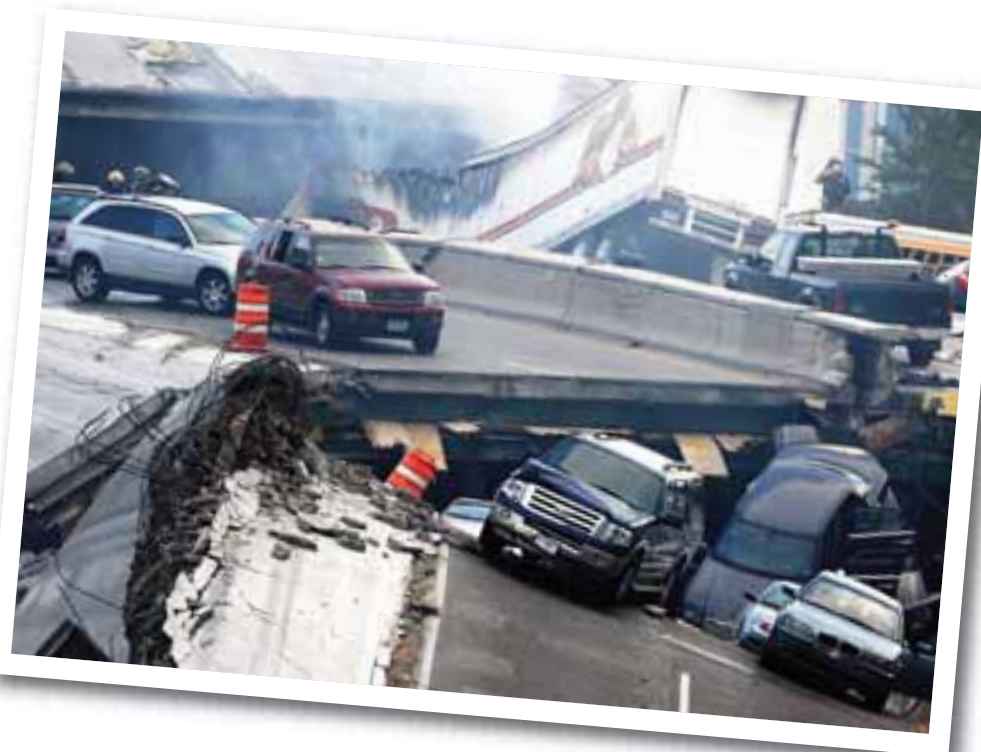
Vehicles are scattered along the broken remains of the Interstate 35W bridge in downtown Minneapolis after the span collapsed into the Mississippi River during evening rush hour Aug. 1, 2007.
