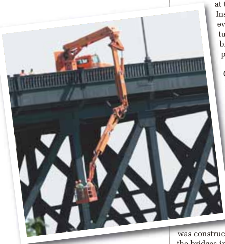
Inspectors use a mechanical arm to examine the condition of New Jersey's 75-year-old Pulaski Skyway. It's an example of the nation's aging infrastructure.
