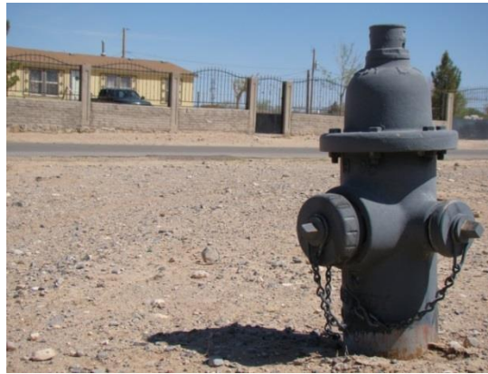
Fire hydrant in Vinton painted black because it is not functional due to lack of pressure.
