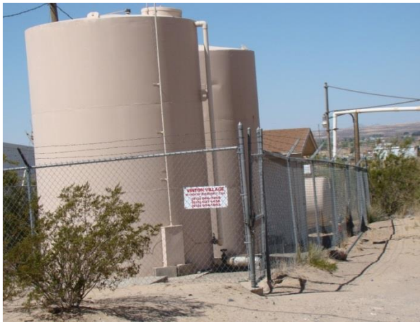
Local well of private provider in Vinton
