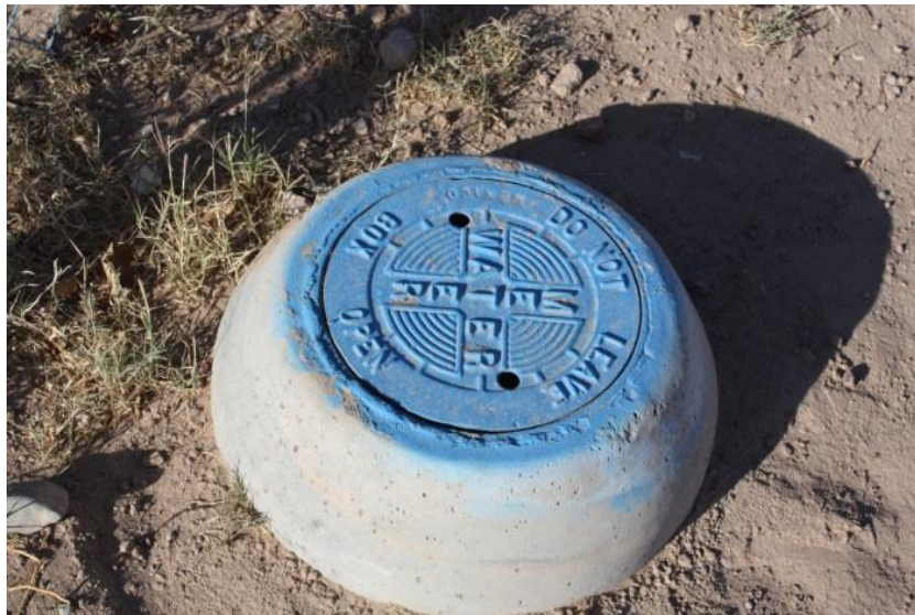
EPWU cover for water meter box
