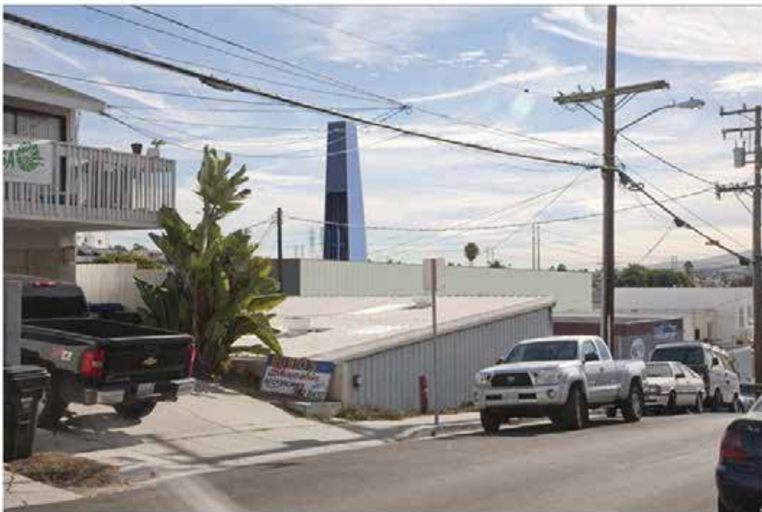
View 18: During Phase 2 with Drill Rig at Well 4
