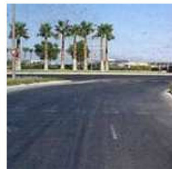
Figure 8: Summerlin, Nevada Roundabout
