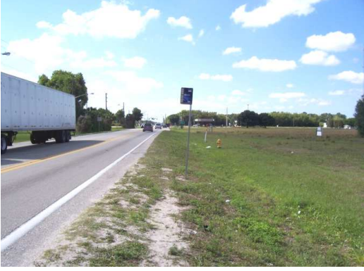
Figure 11: Ortiz Avenue & Lockett Road Bus Stop
