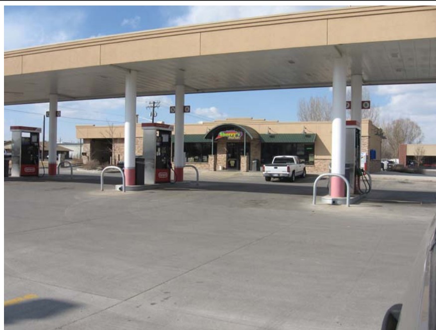
Convenience store on East 24 th Street
