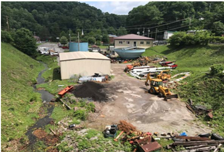
Jenkins Water Treatment Plant looking north from Elkhorn Dam
