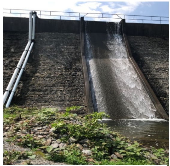
Elkhorn Dam Spillway
