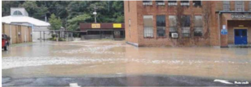
Flooding in 2013 caused $60,000 in damage to McDowell Elementary School in McDowell, Kentucky.
