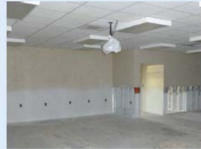
Figure F-6 Wall repair and reconstruction to resist future flood damage. (Photo source: Reynolds Restoration Services, Inc.)
