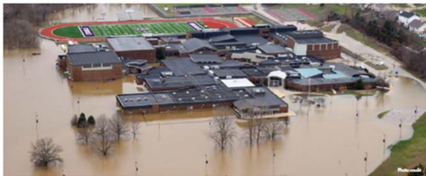
In December 2015, heavy rain flooded Eureka High School in Eureka, Missouri, causing millions of dollars in damage.
