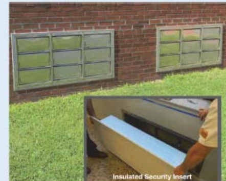
Figure F-8 Flood vents were installed throughout most of the school. Allowing floodwater to enter prevents structural failure of walls if water is outside but not inside (Smart Vent, 2016).
