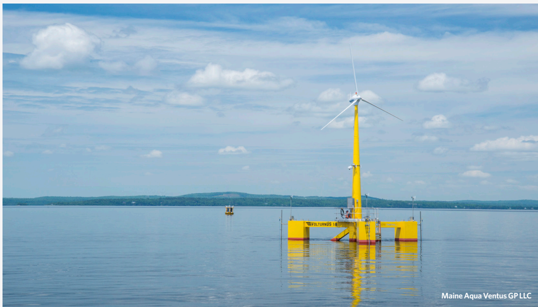
VoltornUS, the nation's first offshore floating wind turbine, off the coast of Castine, Maine.
