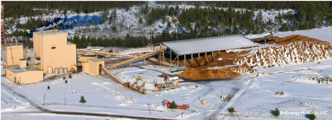
ReEnergy biomass facility in Ashland.
