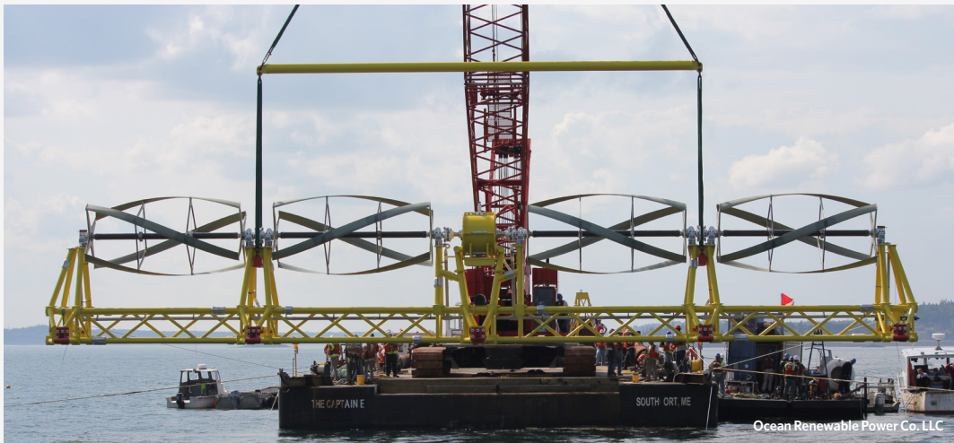
Ocean Renewable Power Co.'s TidGen® Power System prior to installation at the company's Cobscook Bay Tidal Energy Project site in Maine.
