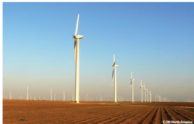
The 782-MW Roscoe wind farm in West Texas
